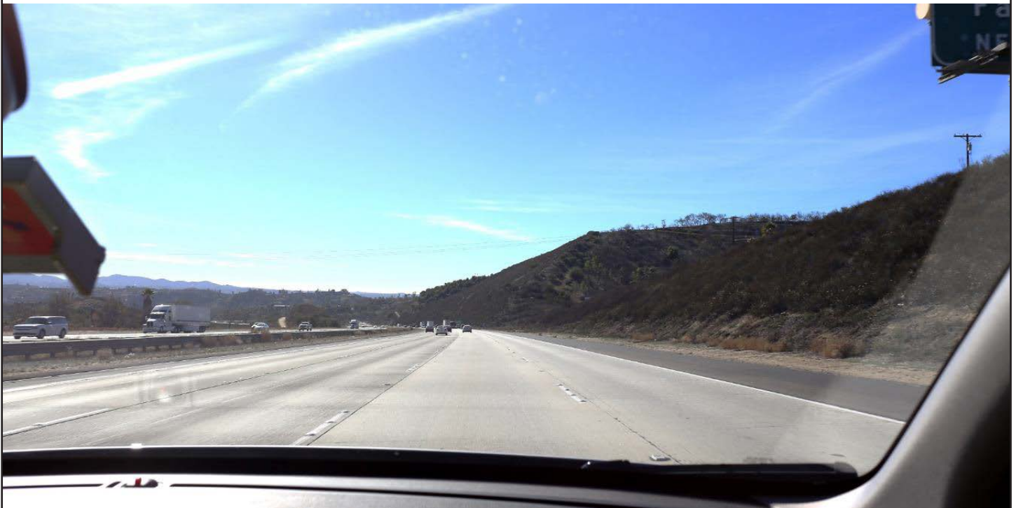
Photograph 4 (LCU 1). View looking south along I-15 near approximate MP 3.2, as seen from a vehicle traveling south along I-15.
