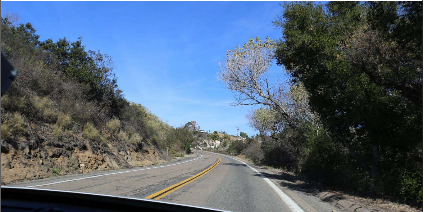
Photograph 16 (LCU 1). View looking northeast along Old Highway 395 near approximate MP 12.1.
