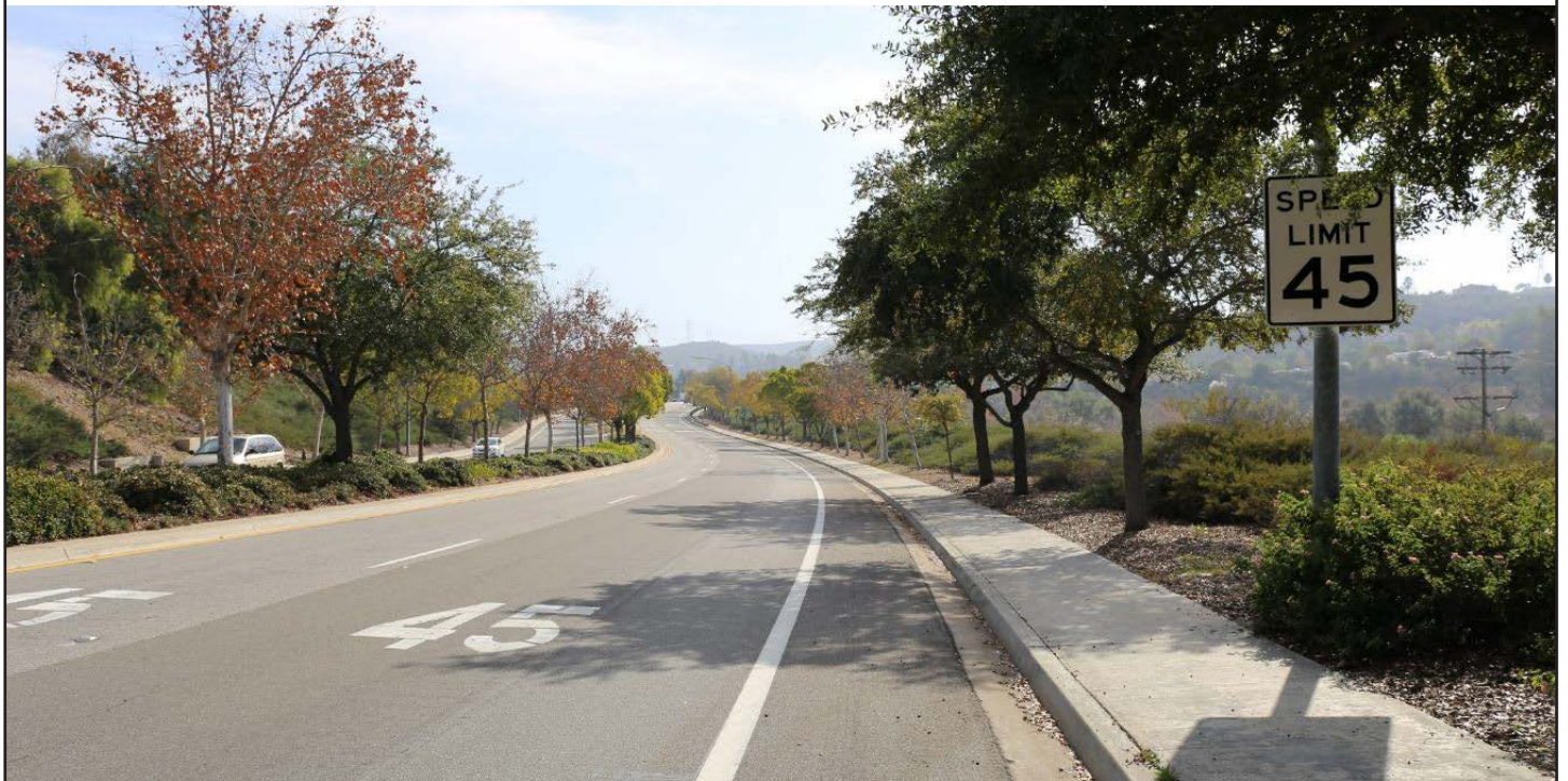
Photograph 32 (LCU 4). View looking south along Pomerado Road near MP 38.9.
