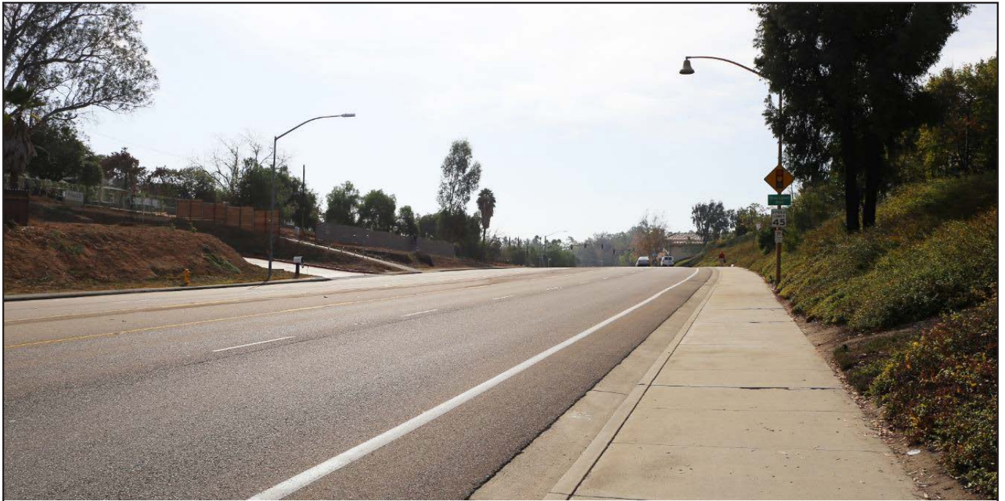
Photograph 31 (LCU 3). View looking south along Pomerado Road near approximate MP 34.0.
