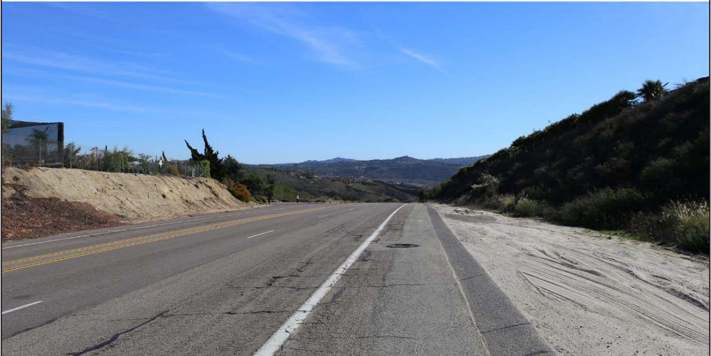
Photograph 12 (LCU 1). View looking southeast along Old Highway 395 near approximate MP 10.8.
