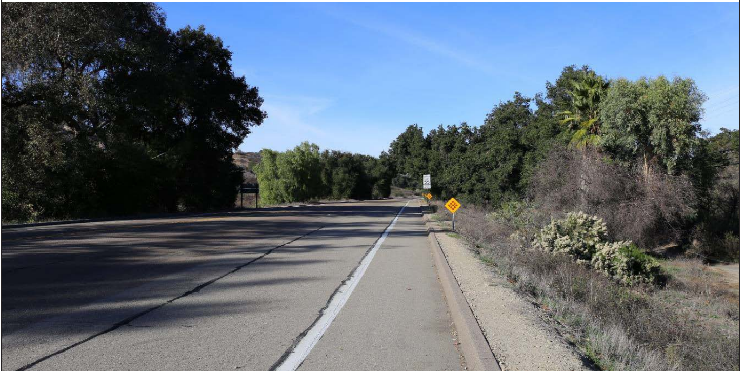
Photograph 18 (LCU 1). View looking north-northwest along Old Highway 395 near approximate MP 15.5.
