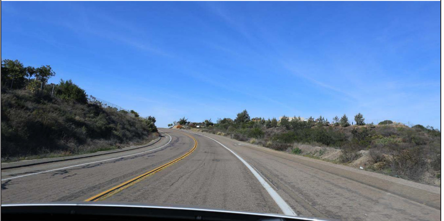
Photograph 14 (LCU 1). View looking northwest along Old Highway 395 near approximate MP 11.0.
