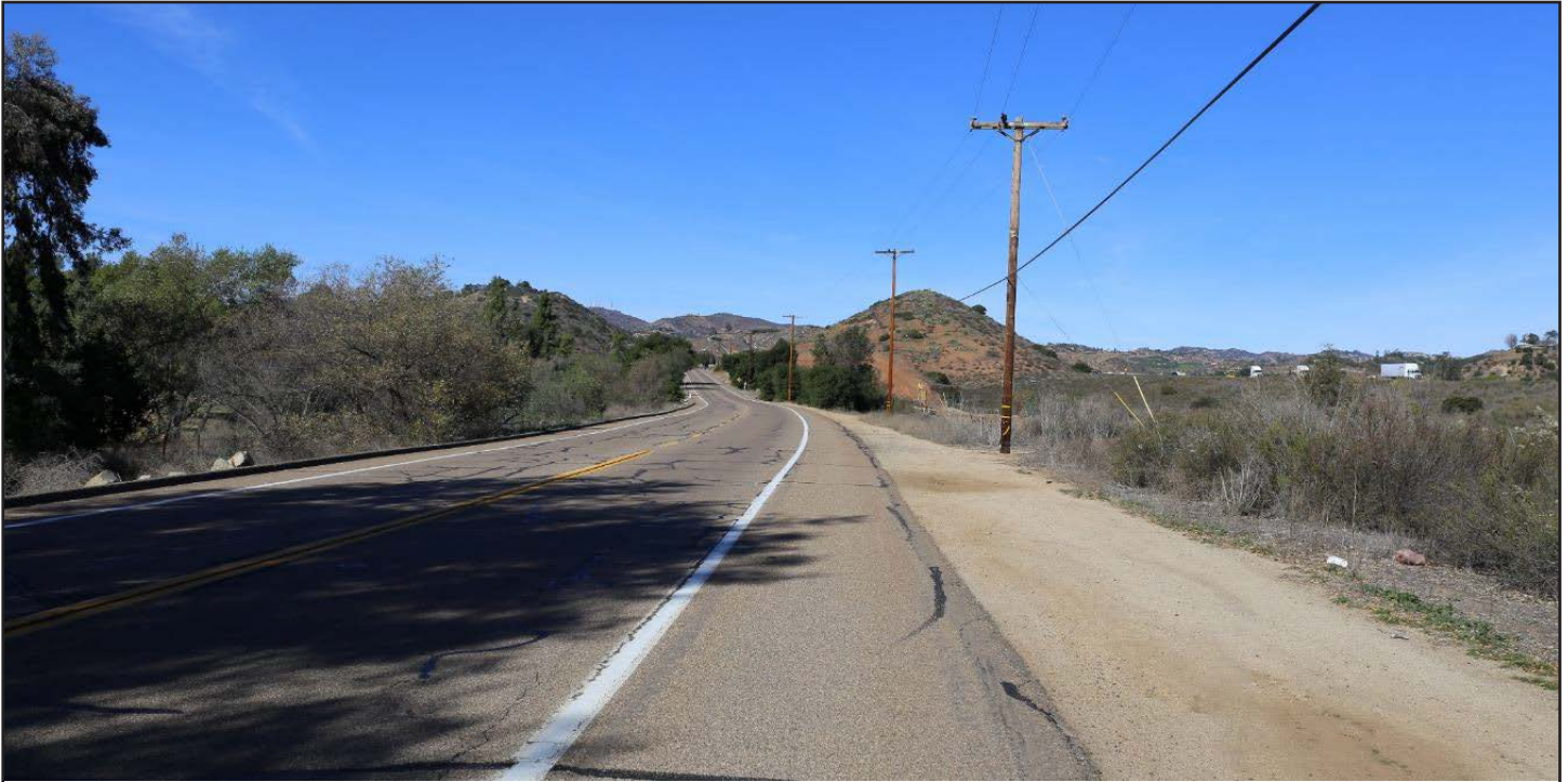
Photograph 9 (LCU 1). View looking north-northwest along Old Highway 395 near approximate MP 6.3.
