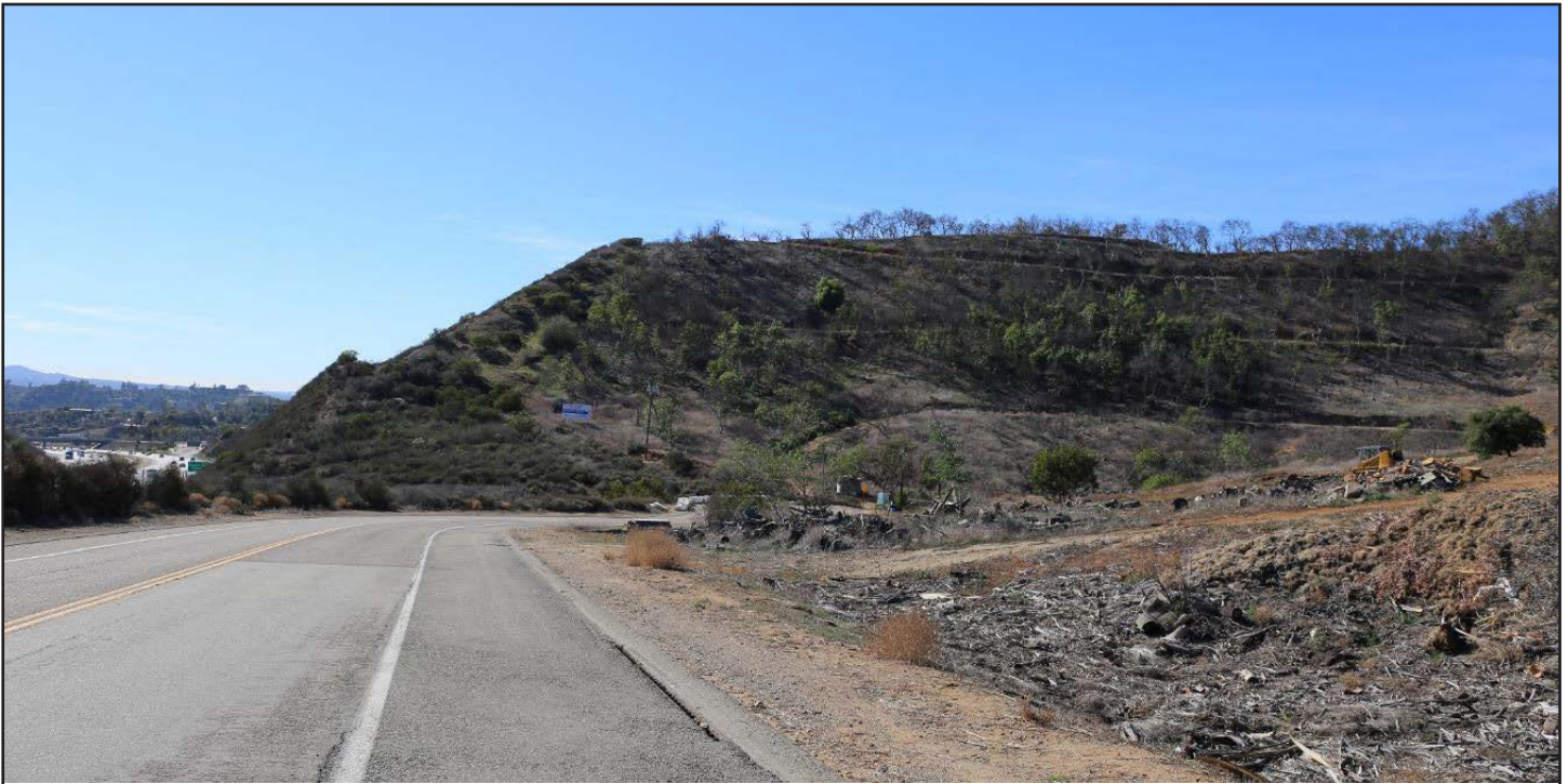
Photograph 3 (LCU 1). View looking southwest toward the proposed Project right-of-way (ROW) from the southwestern end of Rainbow Hills Road at approximate MP 3.2.
