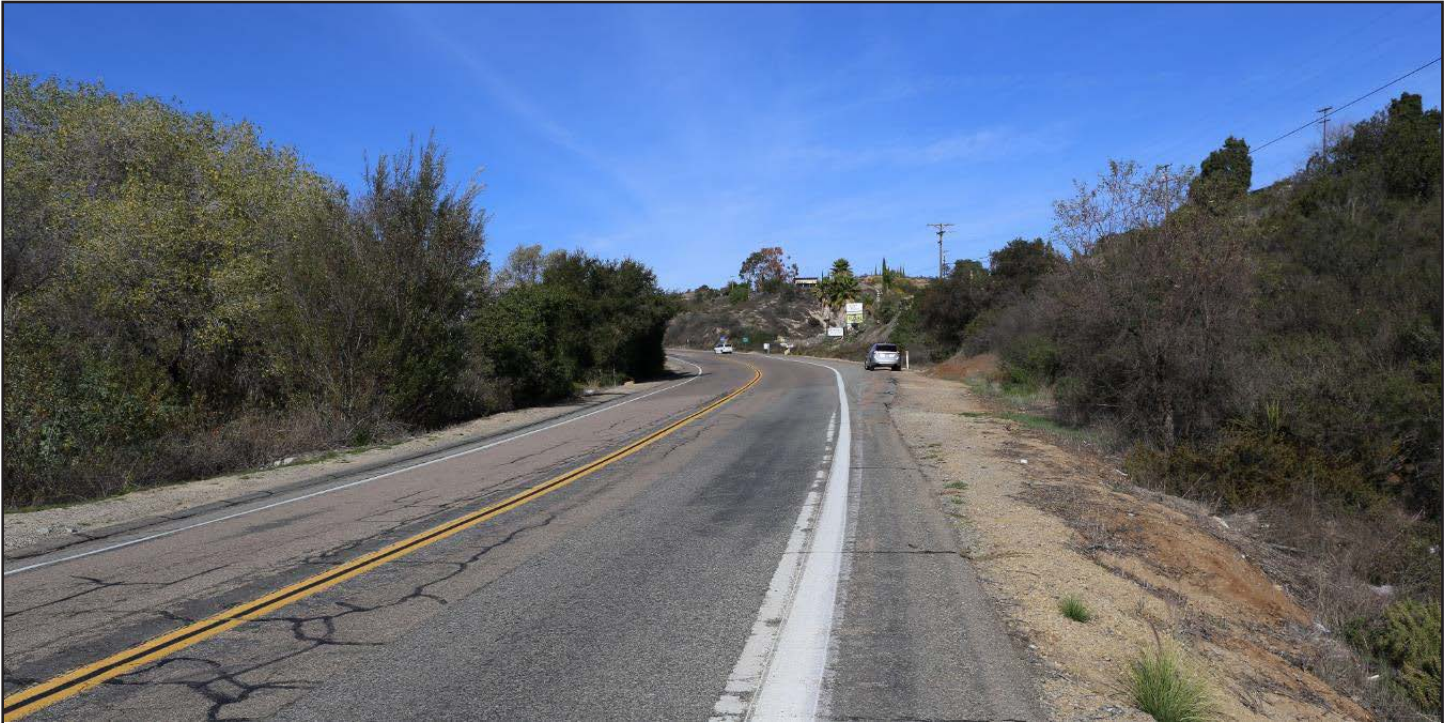
Photograph 15 (LCU 1). View looking northeast along Old Highway 395 near MP 12.1.
